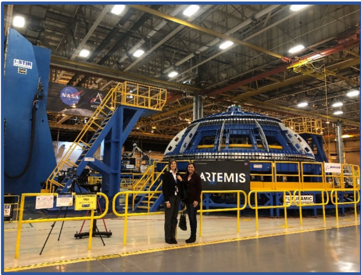
UofM Physics Alumna Michele Wilson (left) in front of the friction-stir welding fixture used to construct the dome ends on the LOX (liquid oxygen) and LH2 (liquid hydrogen) fuel tanks for the Artemis core stage at NASA's Michoud Assembly Facility in New Orleans.
