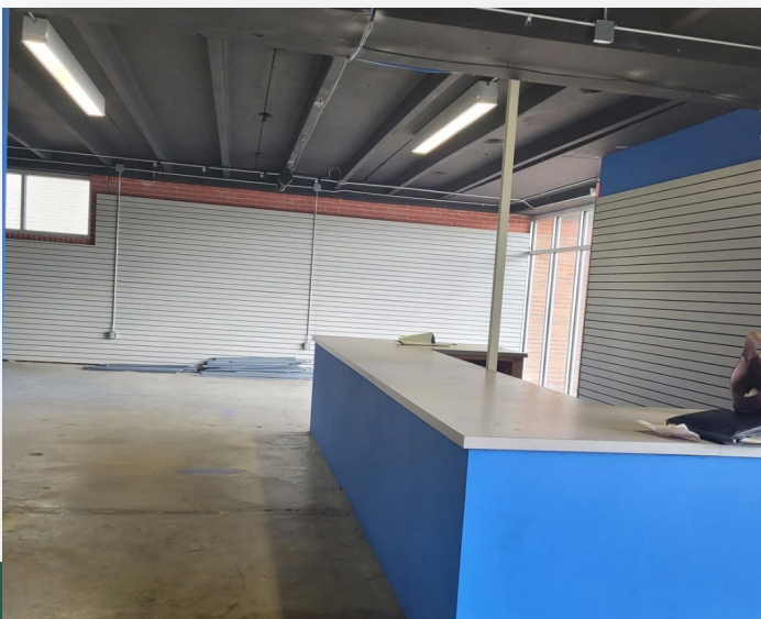
Walker Avenue Site Prior to Renovation
