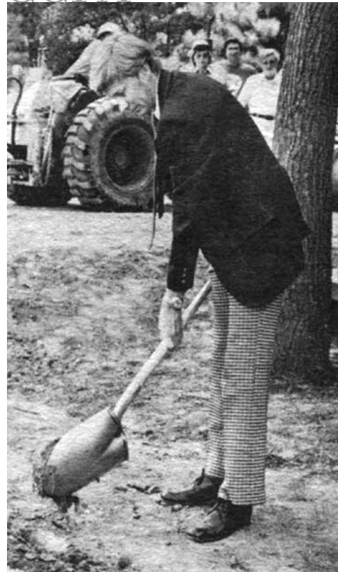
Dean Richard R. Ranta breaks ground on CCFA Building.
